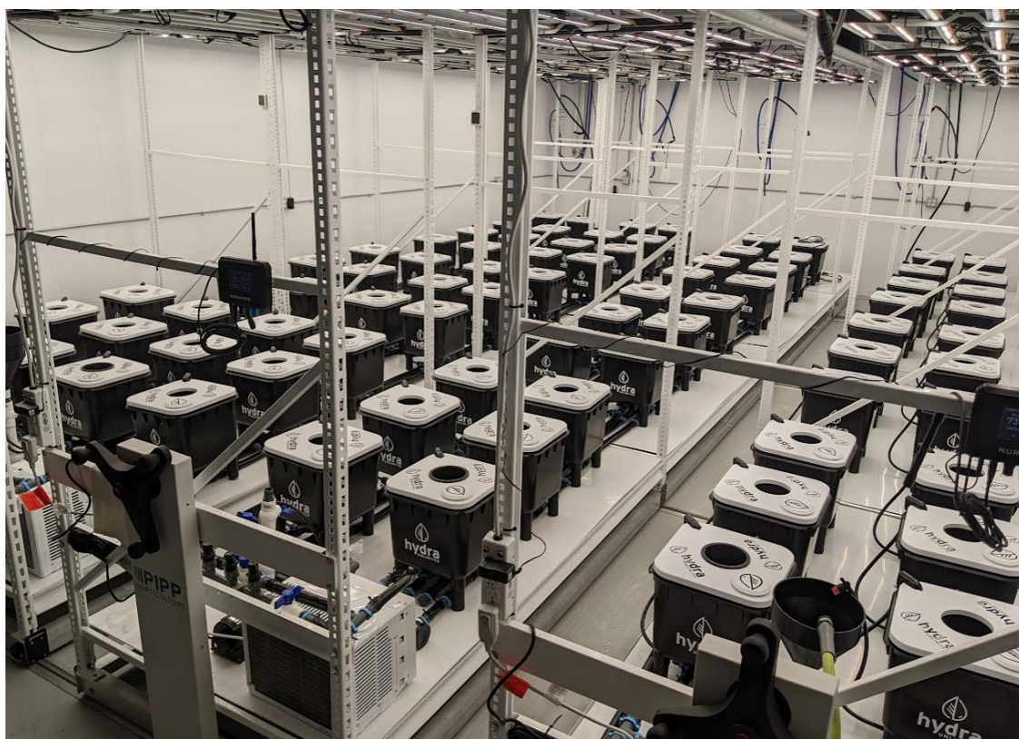
Figure 1: HydraMax systems during setup within grow room at CANNABIS COMPANY
